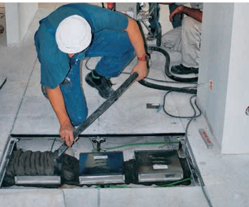
The topic of fire protection is becoming increasingly important. Here, a distribution shaft is being filled.
