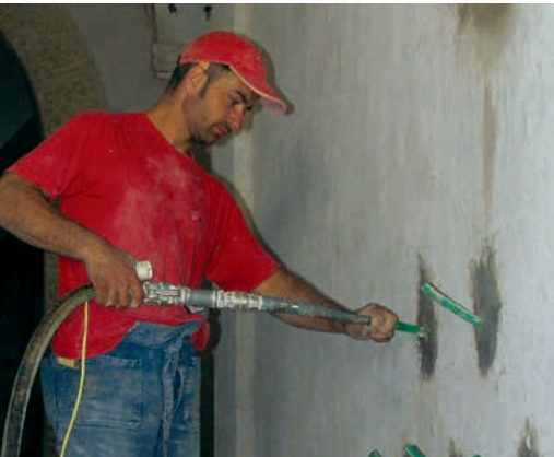
The Sprayboy injecting mortar into the holes.
